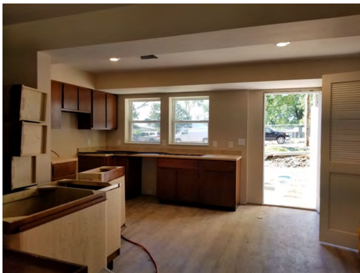
Bldg 8 Unit E Kitchen
