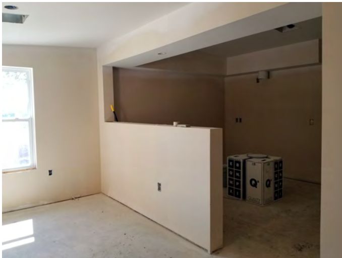
Bldg 9 Unit A Kitchen
