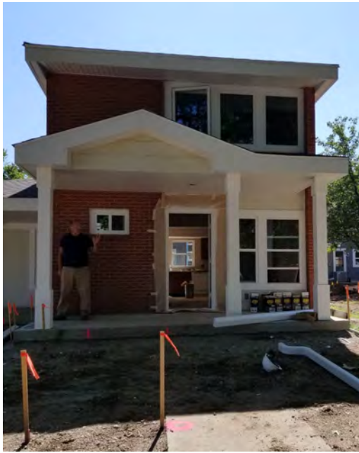
Building 4 Front Exterior
