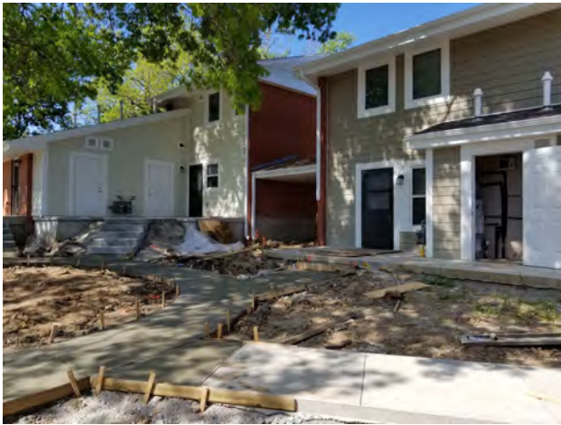
Bldg 6 & 7 Rear Exterior
