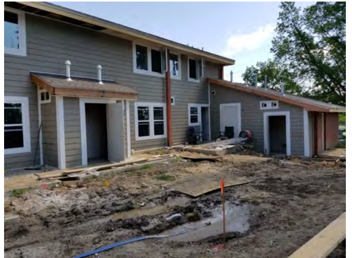
Bldg 9 Rear Exterior
