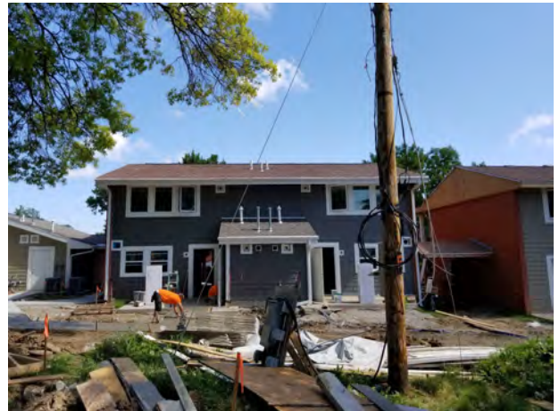
Bldg 8 Rear Exterior
