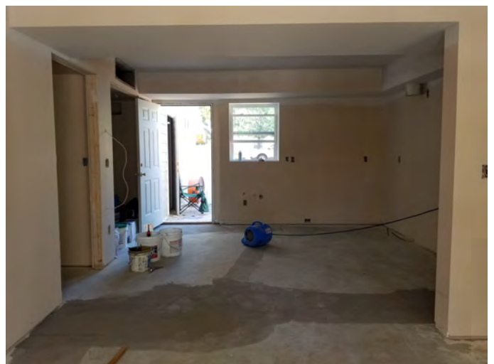
Bldg 9 Unit B Kitchen
