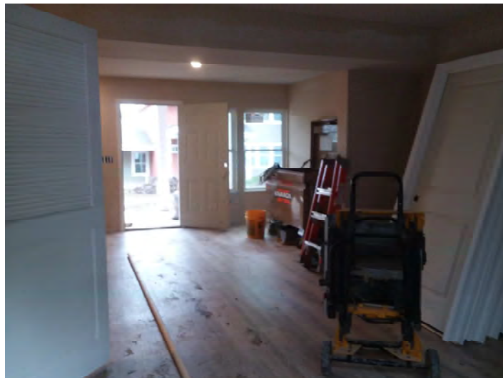
Building 5 - B Unit Interior
