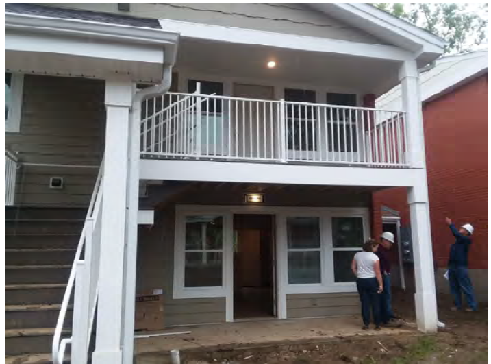
Building 7 - Front Exterior
