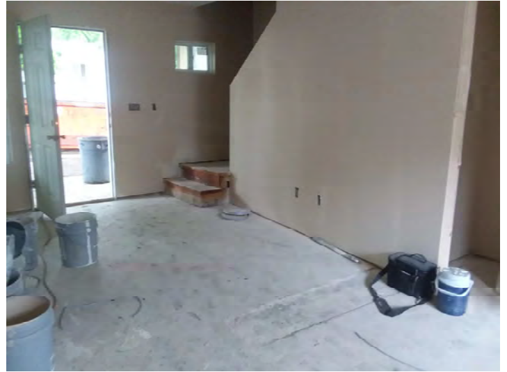
Building 4 - B Unit Interior
