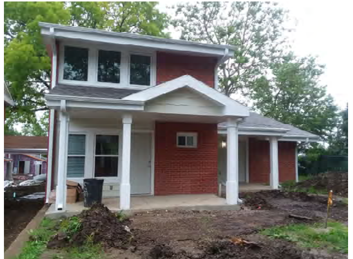
Building 6 - Front Exterior
