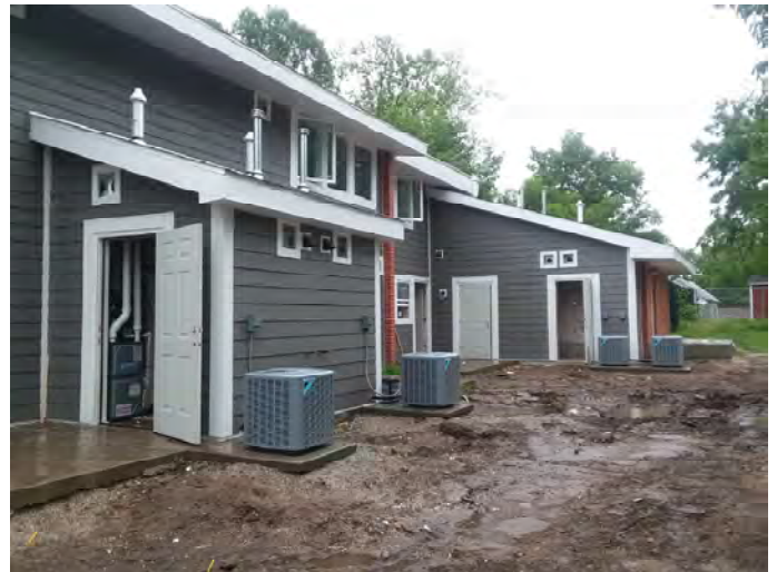
Building 5 - Rear Exterior
