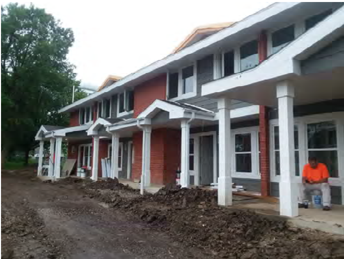
Building 5 - Front Exterior
