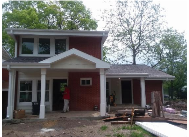
Building 6 - Front Exterior
