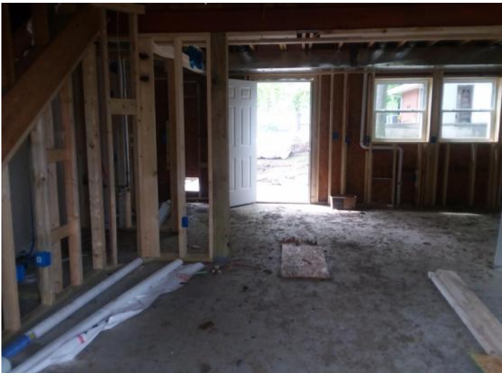
Building 8 - E Unit Interior
