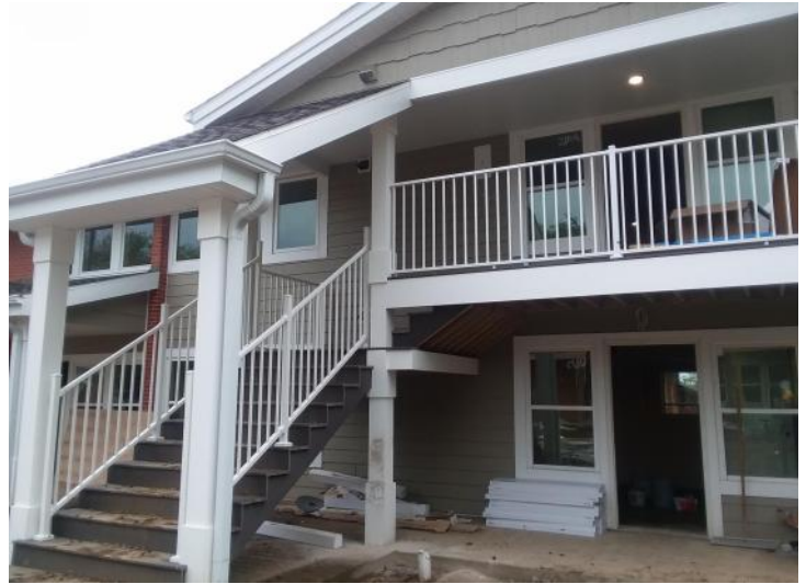
Building 7 - Front Exterior
