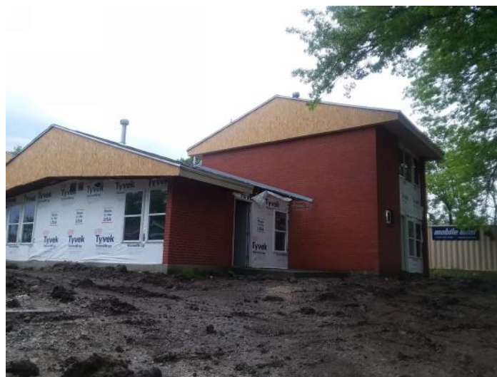
Building 4 - Front Exterior
