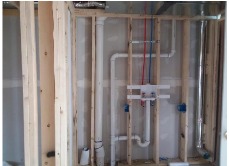
Building 8 - E Unit - Fire-Rated wall separation
