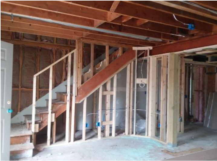
Building 5 - E Unit Interior
