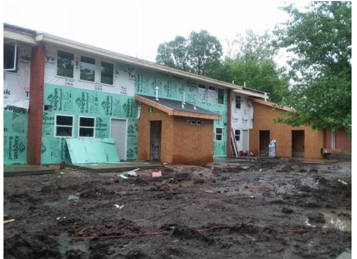
Building 5 - Rear Exterior
