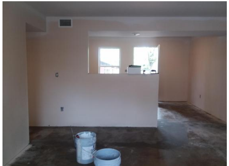
Building 7 - C Unit Interior
