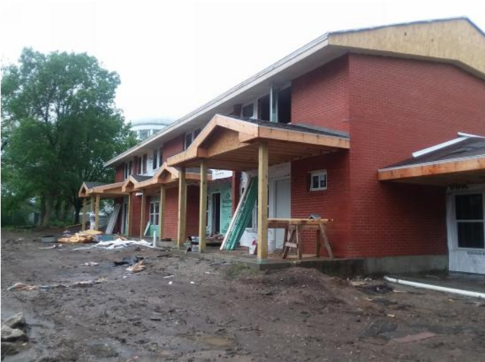
Building 5 - Front Exterior
