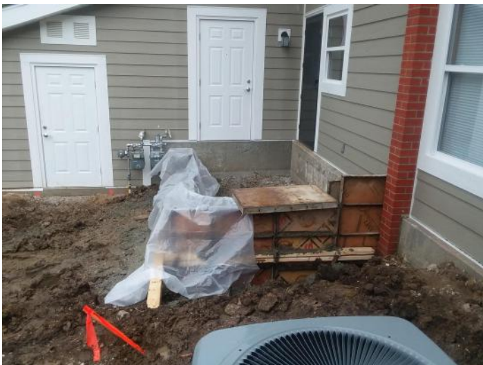
Building 2 B Unit Rear Patio Re-Pour
