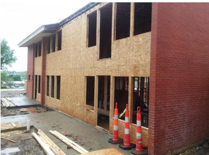
Building 9 - Front Exterior
