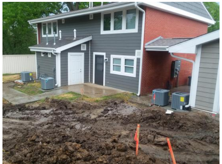
Building 3 Rear Exterior and Site Re-Grading
