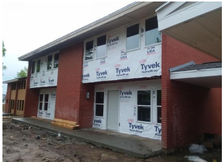
Building 8 - Front Exterior
