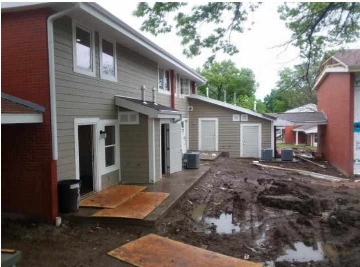
Building 7 - Rear Exterior
