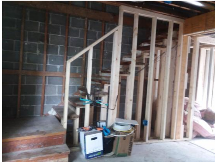
Building 4 - B Unit Interior
