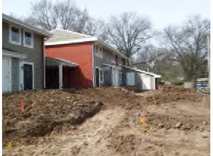
Building 2 - Rear Yard Grading
