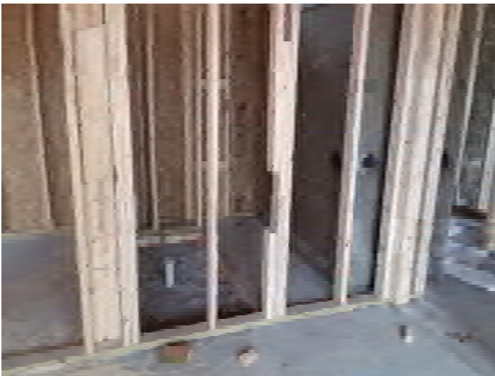
Building 4 - Termite Damage at Landing Beam
