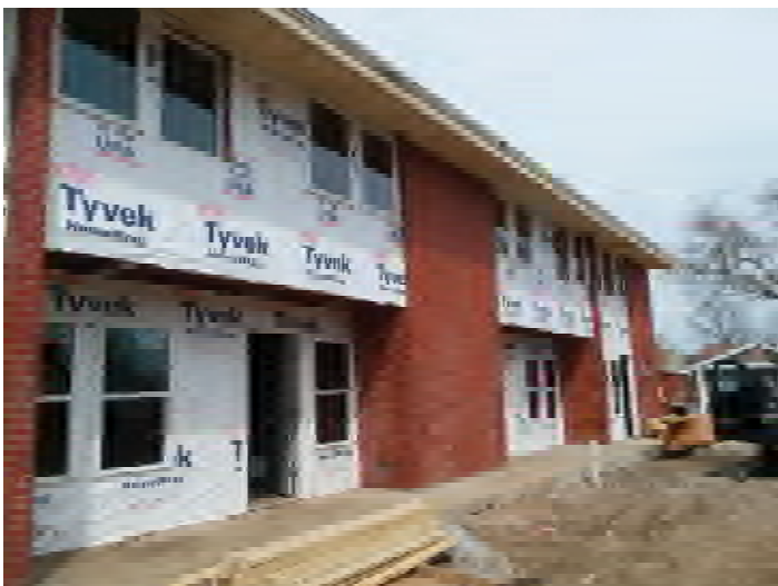
Building 5 - Front Exterior
