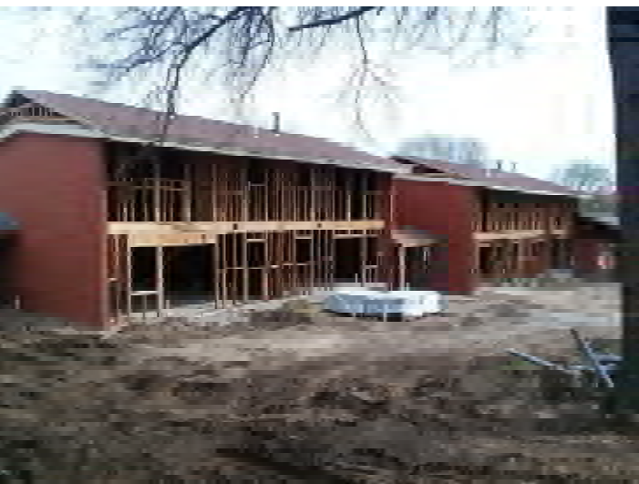
Buildings 8 & 9 - Rear Exterior
