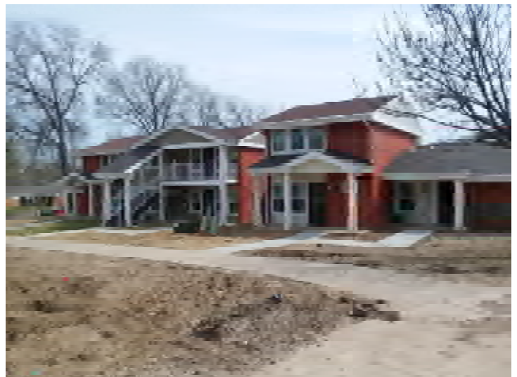
Buildings 10 & 11 - Front Exterior
