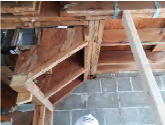
Building 4 - Termite Damage at Landing Beam
