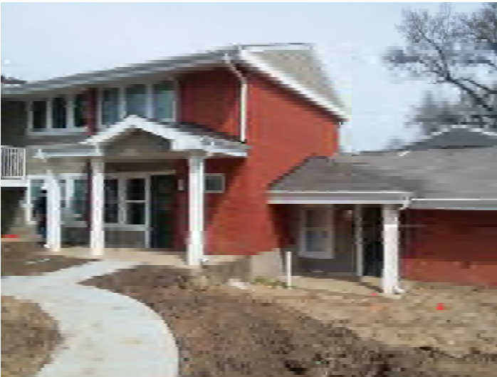
Building 2 - Front Exterior
