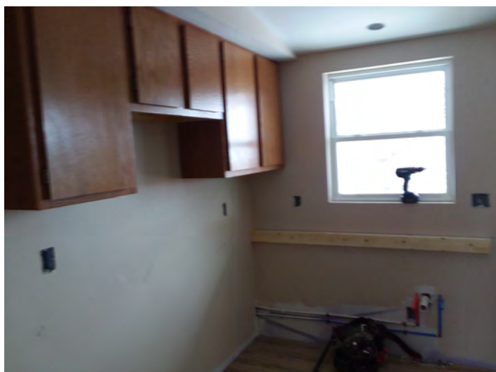
Building 8 D Unit Kitchen
