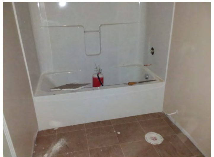
Building 8 D Unit Bathroom
