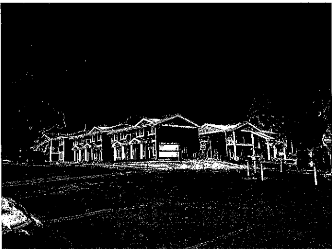
Building 14 & 15 Front Exterior
