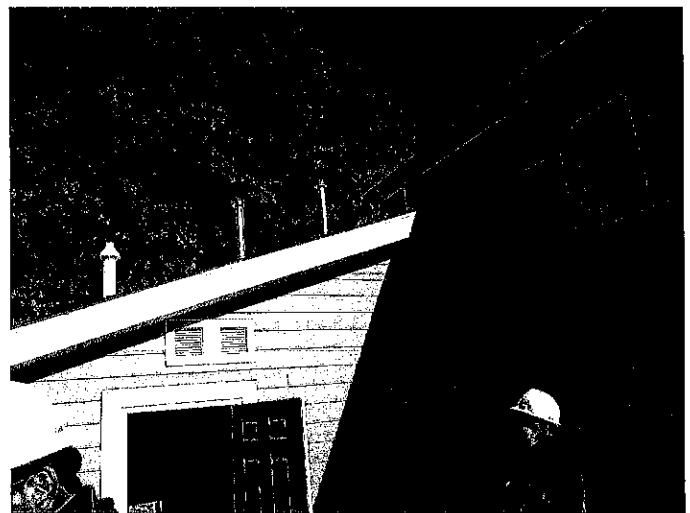
Building 15 Mechanical Closet
