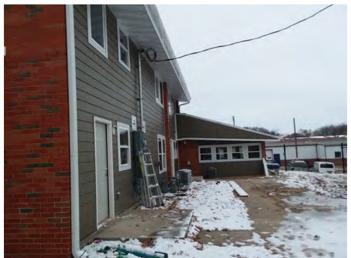
Building 8 Rear Exterior
