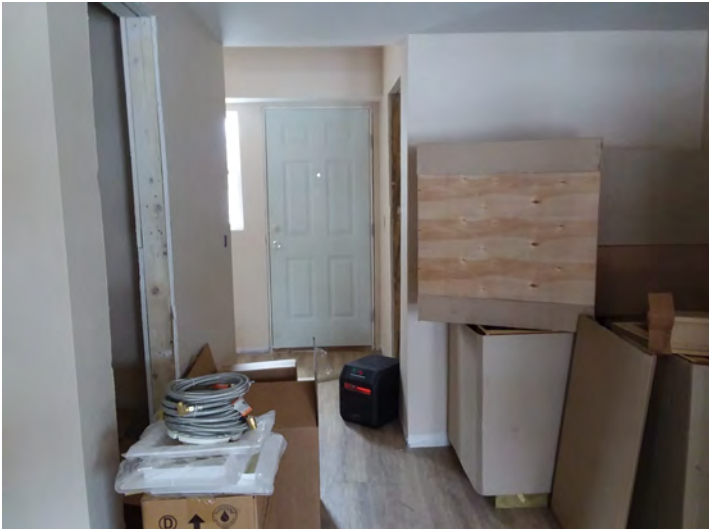
Building 8 B Unit Interior
