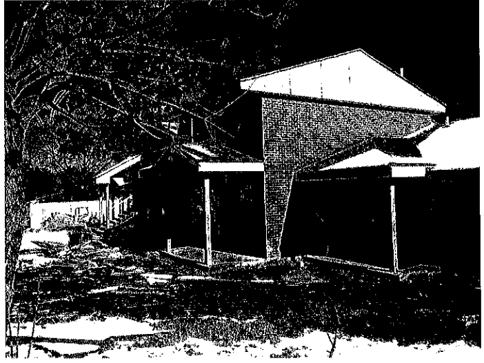
Building 10 - Front Exterior
