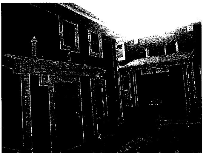
Building 14 & 15 Rear Exterior
