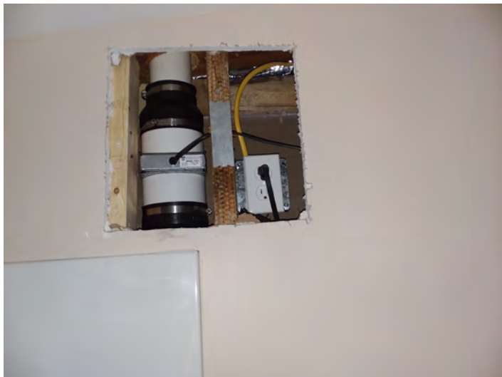
Building 8 C_D Unit Radon Fan
